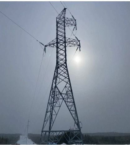
RT064, a dead-end tower (four legged) on line segment RT, on Deer Lake First Nation Homelands
